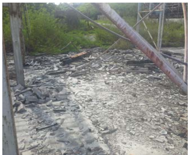
■ Figure 19. Fire-damaged sites often contain significant volumes of ACM debris.
