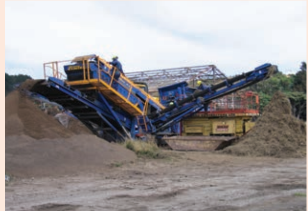
Figure 25. Screening of ACM at Patea Freezing Works site.
