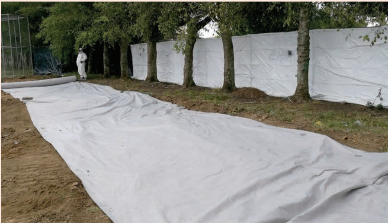
■ Figure 28. Temporary cover of contaminated soil.
