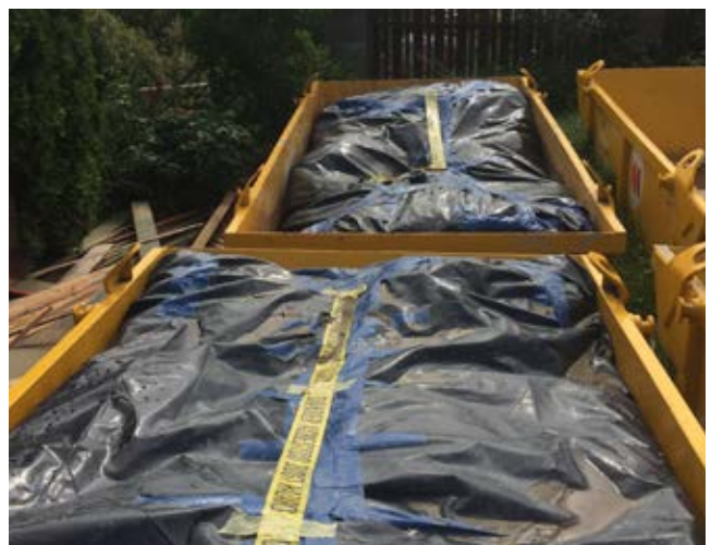
Figure 22. Asbestos-contaminated soil packed and sealed in skips ready for transportation.
