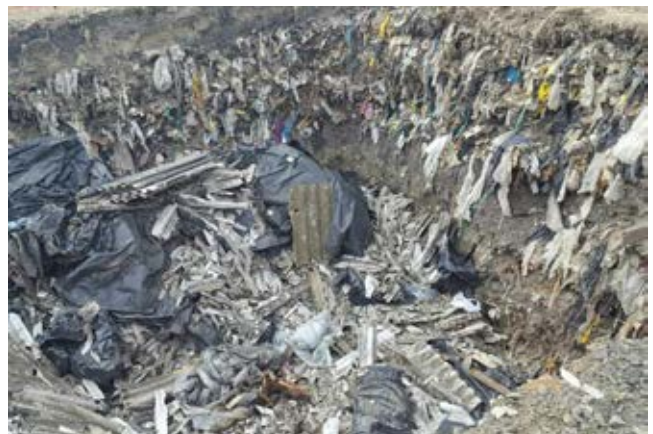
■ Figure 10. Landfill contaminated with a wide variety of asbestos-containing products as a result of dumping demolition waste.
