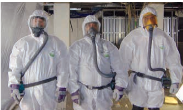
■ Full-face P3 respirators for Class A removal work.
